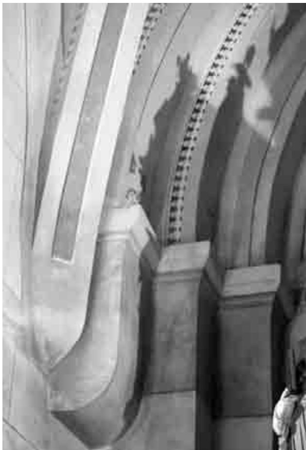
17. Jurklošter, nekdanja kartuzijanska cerkev, iztek reber v severovzhodnem kotu ladje / Jurklošter, former charterhouse church, end of the ribs in the northeast corner of the nave
