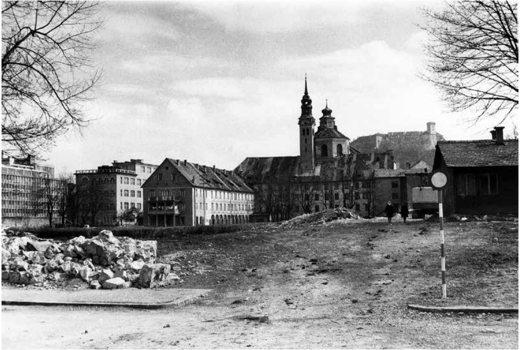
7. The Ursuline convent after demolishing the part of northern wing and western façade of Plečnik's school building before the extension was built
